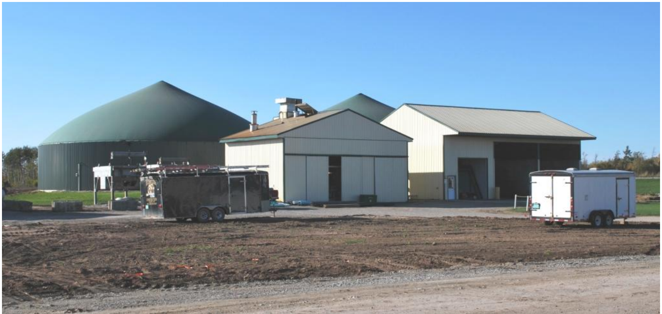
Methane digesters and generator building, Green Valley Dairy, Shawano County J. Moynihan
